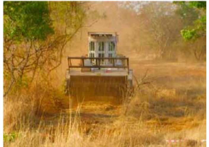
Road clearance operation with the MineWolf
